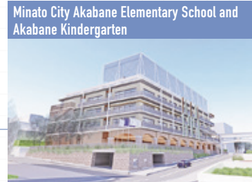
Minato City Akabane Elementary School and Akabane Kindergarten Scheduled start of operation: April 2023 for the elementary school September 2026 for the kindergarten *The completed image is of Akabane Elementary School
