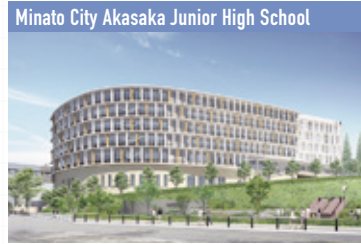
Minato City Akasaka Junior High School Scheduled to begin operation in September 2022 *Will begin operation as an integrated elementary and junior high school in April 2023
