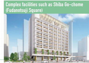
Complex facilities such as Shiba Go-chome (Fudanotsuji Square) Scheduled to open in April 2022
