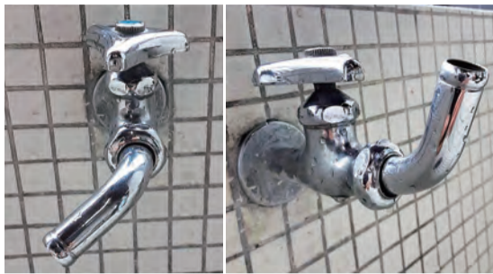
A faucet with a rotating spout which Watanabe submitted as a utility model before joining the Navy. It is still in use today at the Takanawadai Elementary School.
