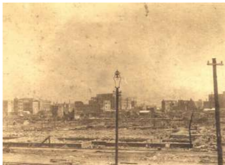
Photos from the Great Kanto Earthquake: Burned ruins in front of Tokyo station, looking towards Nihonbashi (Japan Meteorological Agency website)
