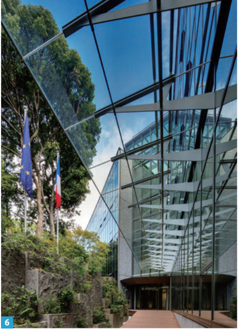
Appearance of the current French Embassy in Japan (Copyright: KAWASUMI Architectural Office)
