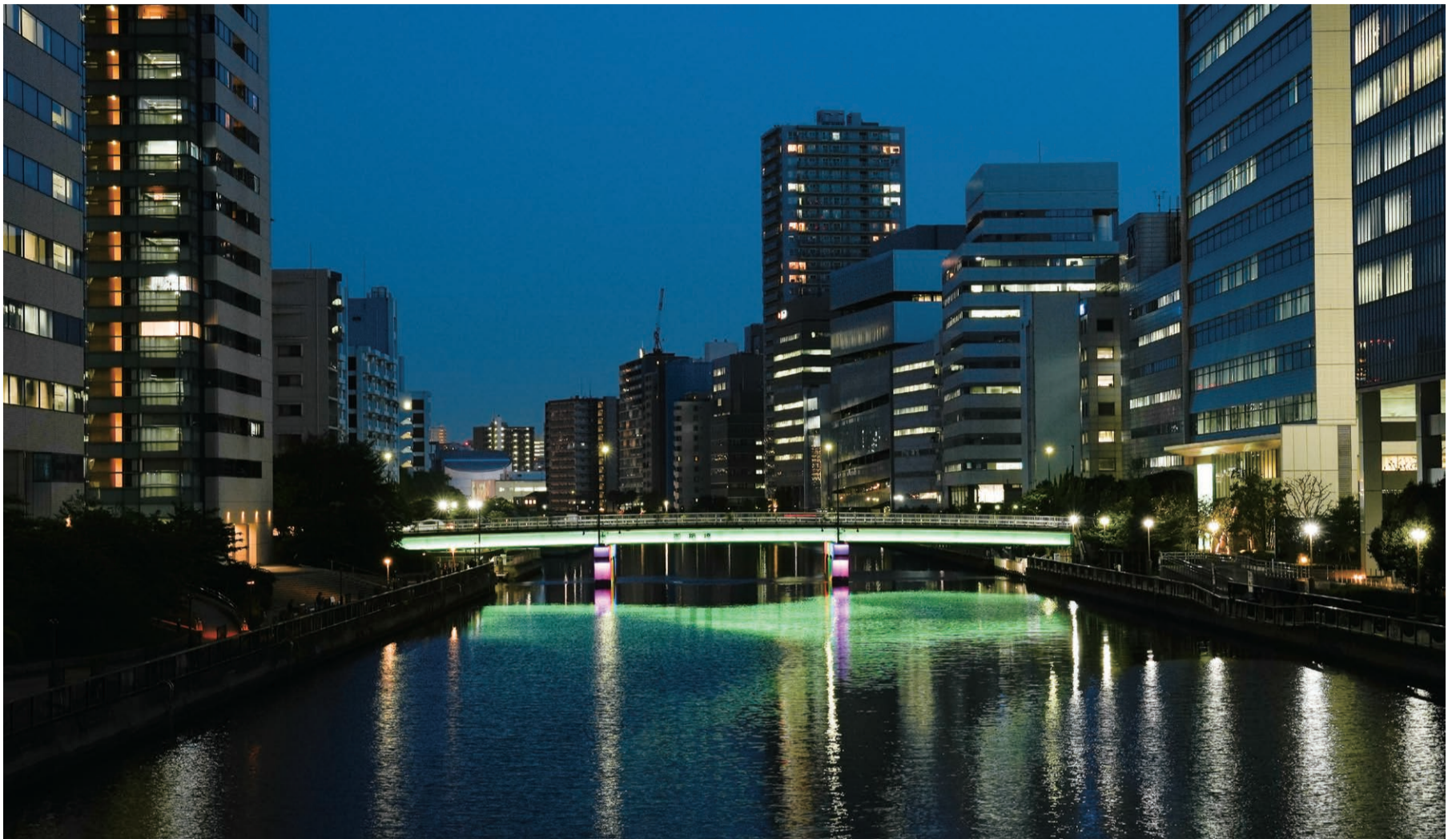
Lighting up of Mitate Bridge, 2-13 to 4-1 Konan Lighting up may be cancelled due to COVID-19 infection prevention measures. For the latest information about the lighting up schedule, please visit the Minato City web.
