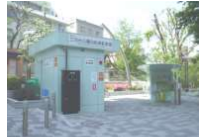
▲Automatic underground bicycle parking
