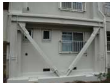
▲Cross braces for earthquake resistance
