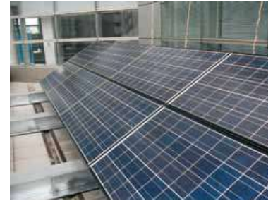
▲Solar power system
