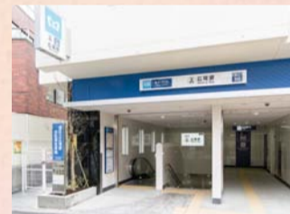
Newly Constructed Exit No. 4
