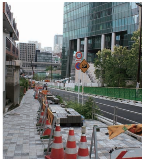
In 2016, it feels more spacious overall. In days of old, the spare house of the Soma Domain could be seen from here.
