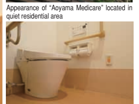
Emergency buzzer is provided at the foot of the resident that can be reached even when the resident gets sick.
