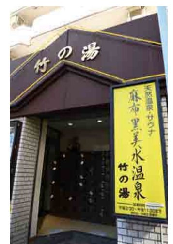
The shoe cupboard and lockers by the entrance are shared making it easy for the customers.
