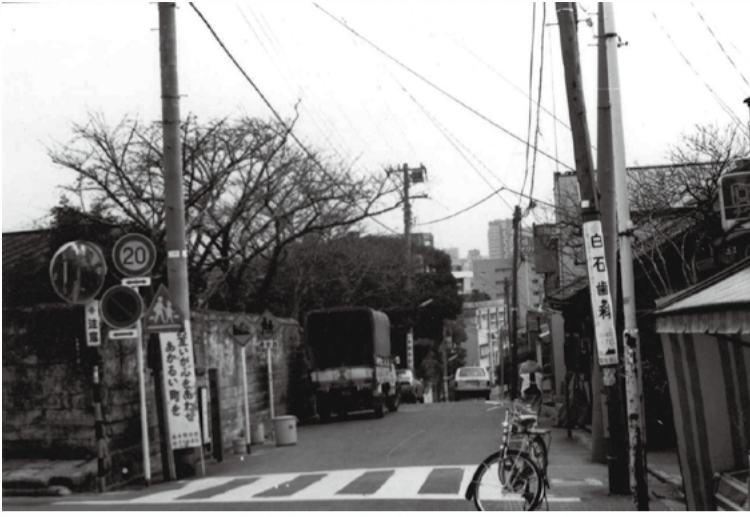
1975: Yakuen-zaka Slope from on top of the slope. Photographed taken by Masanori Taguchi and provided by Shigehisa Taguchi
