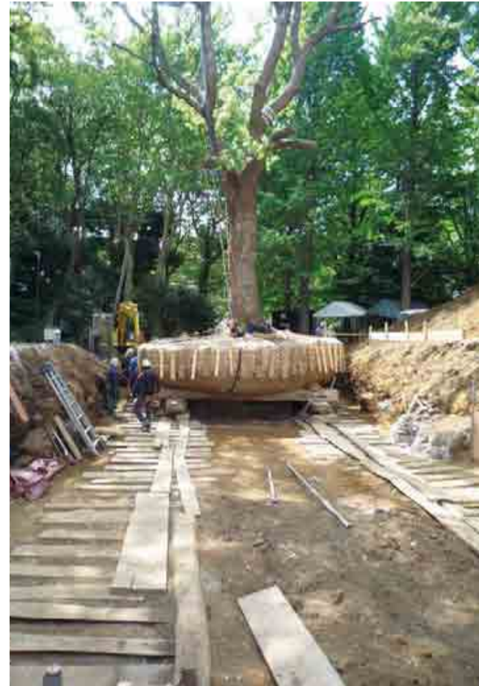
The afternoon of the day the transplantation started. The tree finally arrives at the landing platform. The trajectory is adjusted with the koro in front and michiita. After this, the part inserted below the grid-like table is detached and the soil is backfilled the next day.
