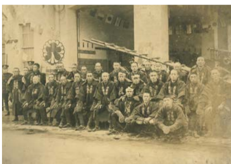
Matoi with the Members (Tobi: Construction Workers) of the Unit No. 6 in Zone Two
