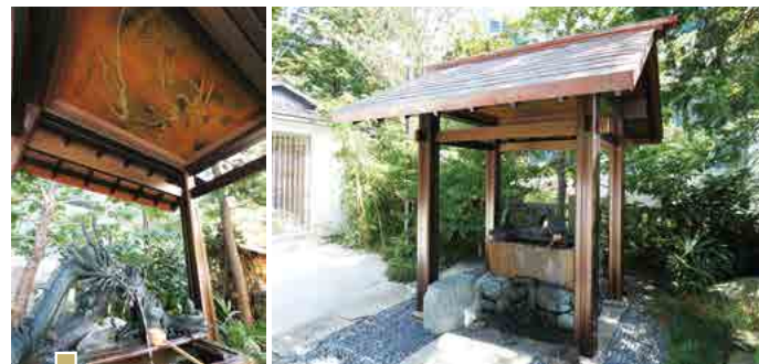
This "Temizuya" (water ablation pavilion) is located on the front right side of Goshaden (the main shrine building). In the water basin, a bronze dragon spouts water. This dragon is quite a dynamic figure, and looks just like the dragon drawn on the ceiling you see going down there. This bronze dragon was offered by the son of a carpenter who was involved in the construction of the shrine in 1957. It was made in Kyoto by special order for this shrine.
