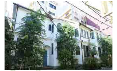
Building No. 4 was listed as a registered tangible cultural property by the Agency for Cultural Affairs on March 29, 2019.
