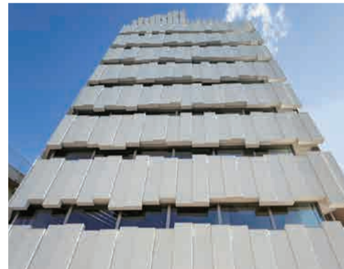
Outer wall ALC panels arranged unevenly This technique is called "yamato-bari" and has been used for a long time on walls in Japan.
