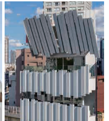
The ALC panels of the outer wall stretch further towards the sky from the top floor.
