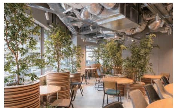
Intentionally exposed ducts on the ceiling increase the impression of height and openness.
