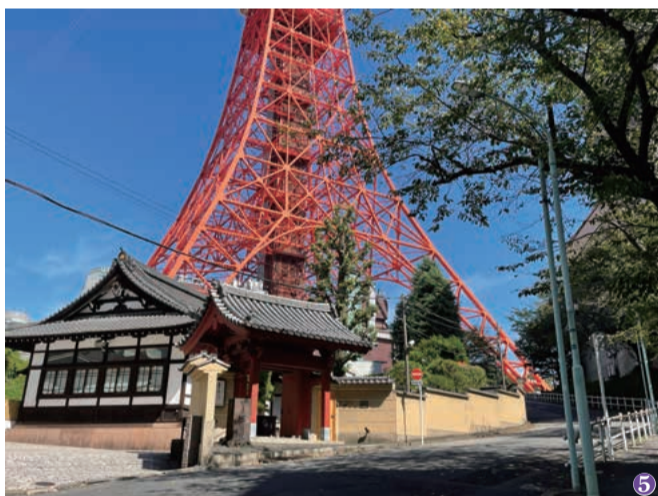
Shinkoin Temple is located adjacent to Tokyo Tower. Tokyo Tower is on a cliff top, while the Temple is below the cliff.
