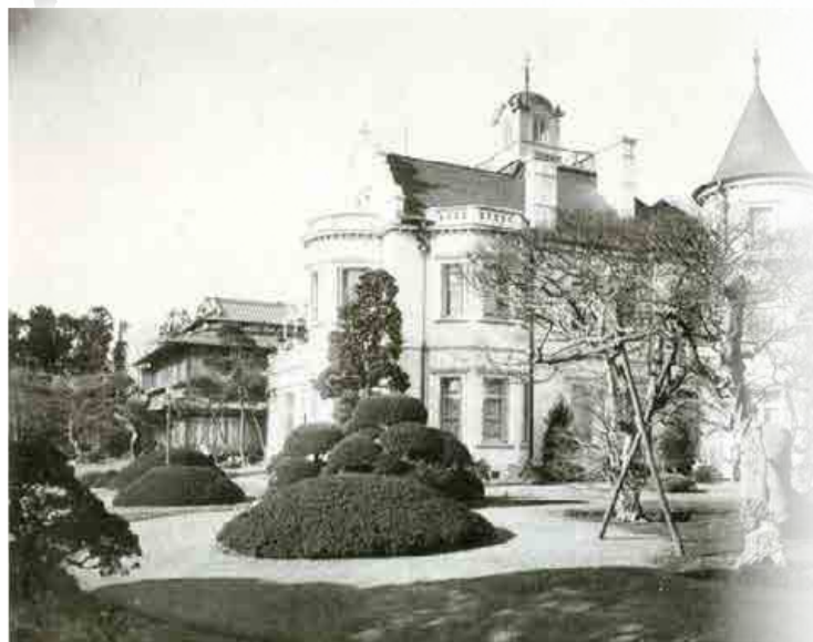
View of both buildings from the east side of the garden
