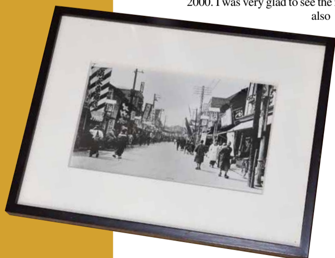
View of Azabujuban Shopping Street in 1913 The Sunaga Gofukuten banner-flag is visible on the front left.
