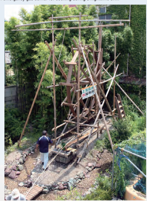
Digging the well with the cooperation of regional residents
