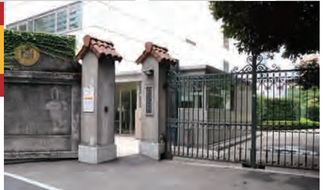
The Spanish colonial gate. The Embassy building is the one on the left and the Ambassador's residence is on the right, behind the garden.
