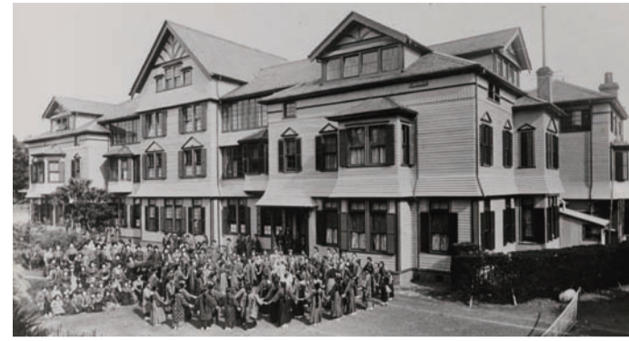
The school at the time Hanako was a student there A wooden four-story building with a floor space of 650 tsubo (2,149m 2 ) (including attached buildings), the school is an impressive structure. The school building connects to living quarters for the western teachers. On the first floor are classrooms, a dining hall, the principal's office, and the teachers' room. The second and third floors house dormitory rooms for boarding students and on the fourth floor there is a prayer room. Hanako lived in a room on the second floor with several other students. At that time, the school had around 200 students, with approximately half of them boarders and half day students.
