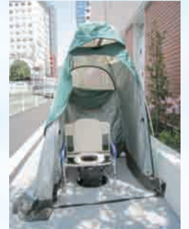
The manhole diameter is small, only 20cm, in order to prevent small children from falling in. The cover cannot be opened without the use of a special tool. The level of comfort of the toilet is more than adequate, and very stable. (In front of Azabu Nursery School).
