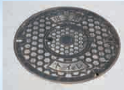
The manhole diameter is small, only 20cm, in order to prevent small children from falling in. The cover cannot be opened without the use of a special tool. The level of comfort of the toilet is more than adequate, and very stable. (In front of Azabu Nursery School).
