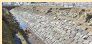
Stone wall on the sea side*
